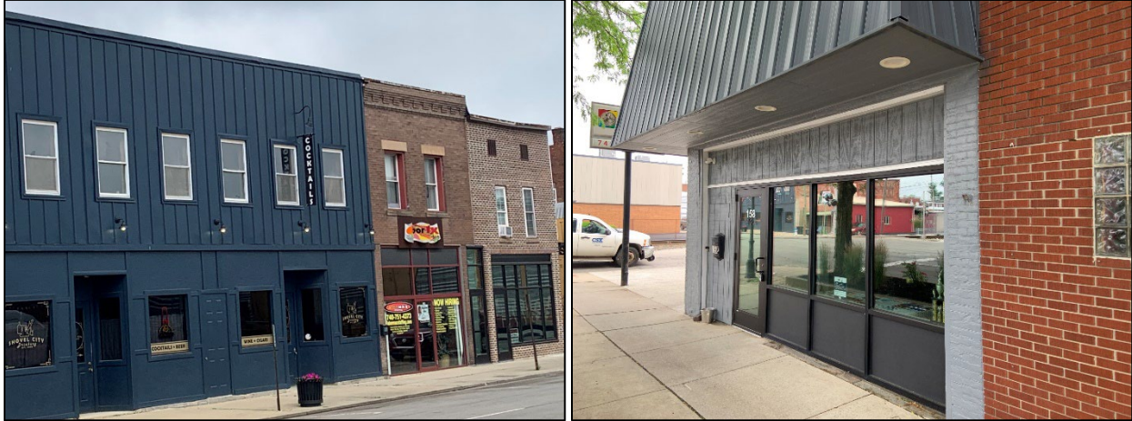
Figure 5 (L): 181 N. Main St. Good: ground floor windows and doors create rhythm; vertical elements in ground floor; separation between storefronts. Not So Good: Siding on upper floor; windows too small; no lintel or sill on windows; no cornice; no transom; no signboard. Compare to building next door with nice cornice and simple details on windows.
