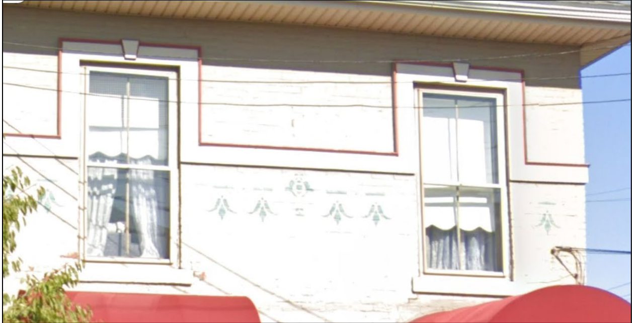
Figure 9: 288 E. Church. Owner used commercially available wood trim, paint, and stencils to return designs of lintels/cornice to a residential structure.
